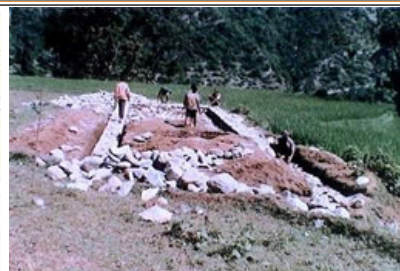
And the foundation is being laid down
