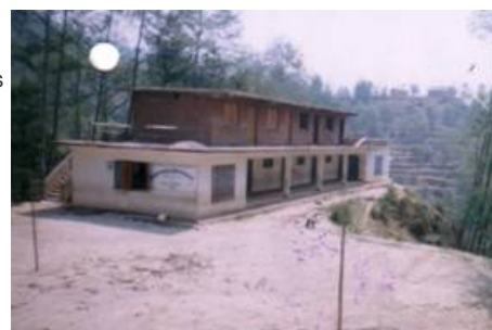
(After) Slab ceiling complete
