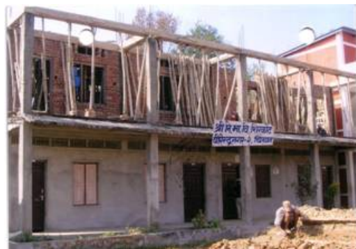
Under construction-Sri Ni Ma Bi School
