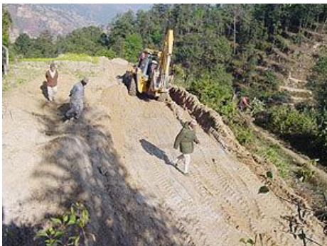
Land Leveling at CIC shelter site in progress
