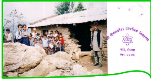
Gogan Dada school in dilapidated condition
