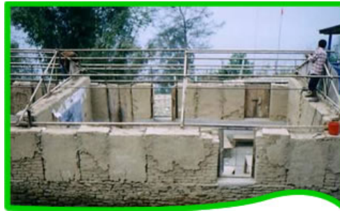
School being reconstructed
