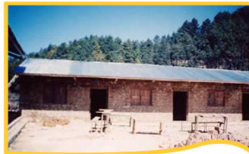
School undergoing reconstruction
